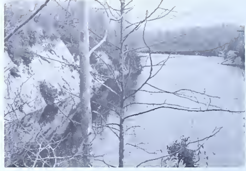
Limestone quarry along Spring Creek in Hershey, Dauphin County; in 1886, the Zimmerman quarry.
